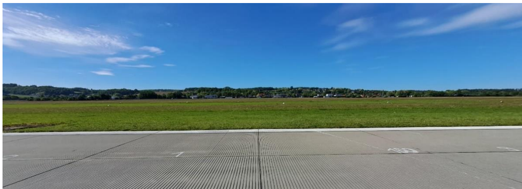
Fig. 2. Example of marking plates (source: own materials)
